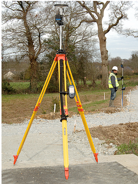
Fig 1. ProMark3 RTK Base/Rover System deployed in the field
